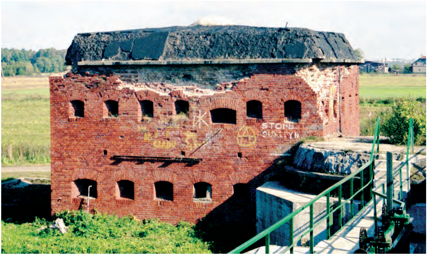
Bergfriede (now: Barkweda, PL) bridge tower
